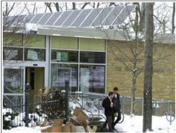
The solar panels installed on the roof of the Fred Landon branch library can be seen from Wortley Road. The solar panel initiative is a partnership between the City of London, Old South Community Organization and the London Public Library. (Sue Reeve, The London free Press)
